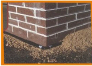
AROUND BUILDING PERIPHERY
